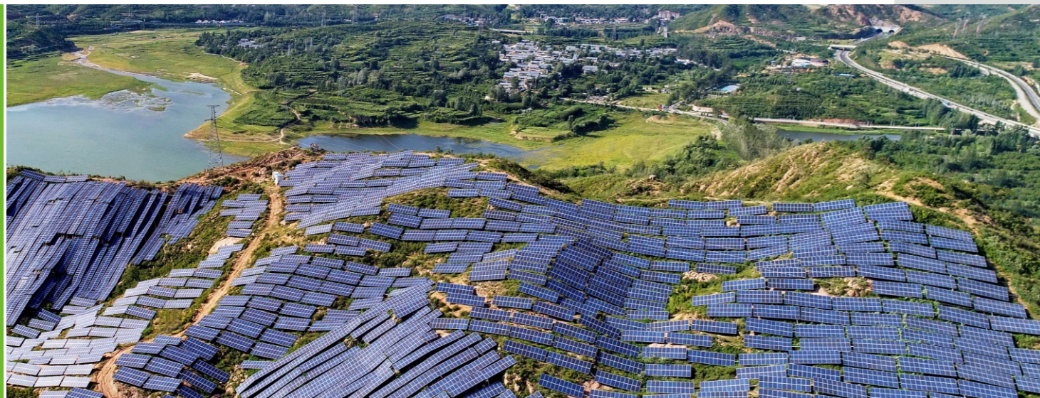
Connect the photovoltaic panel on site
