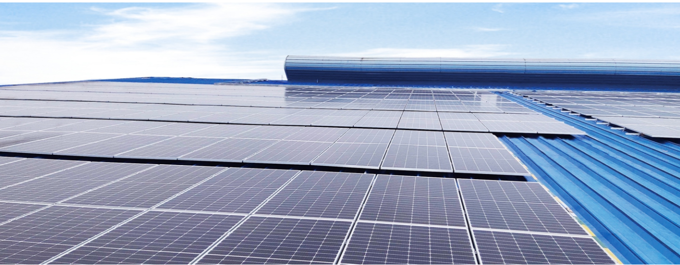
Field wiring connection
